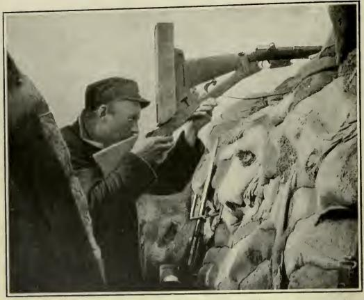
A RIFLE WITH PERISCOPE ATTACHED, So that it can be aimed without exposing the firer.
